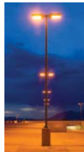
Figure 3.16 The sodium used in this street lamp was generated through the decomposition of sodium chloride. The yellow glow is characteristic of a sodium vapour lamp.
