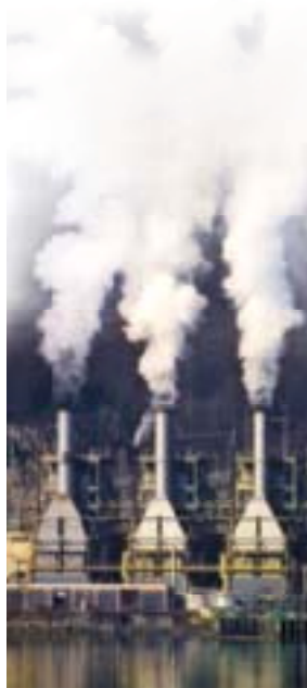
Figure 5.12 Power plants have developed the technology to “scrub” emissions, such as sulfur dioxide, out of the exhaust, using chemicals such as calcium hydroxide.
