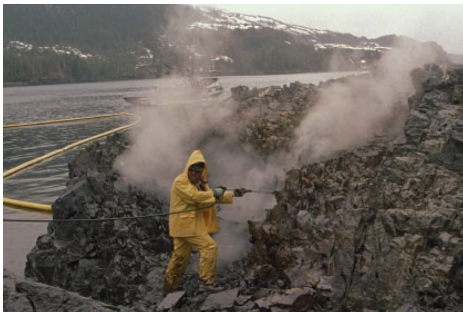
Figure 6 High-pressure steam was used to wash crude oil from the Exxon Valdez spill off the rocky coastline of Prince Edward Sound, Alaska, in 1989. More than 40 million litres of crude oil was spilled.
