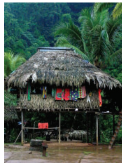
Figure 2 A thatch roof, constructed of palm leaves, can be destroyed by caterpillars. These caterpillars are normally preyed on and controlled by wasps.
