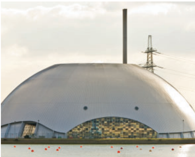
Figure 1 Modern energy-from-waste facilities use garbage to generate thermal and electrical energy.
