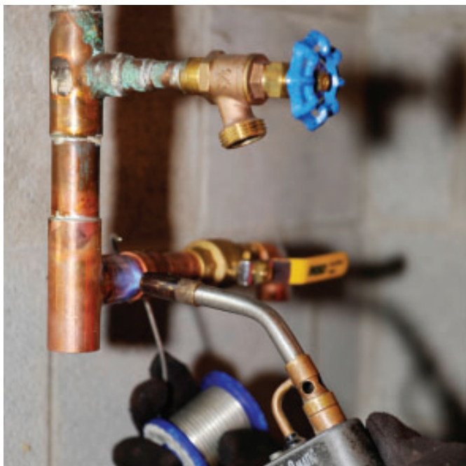
Figure 6 A blow torch is used to melt solder. Lead-free solder consists of non-toxic metals such as tin, copper, and silver.
